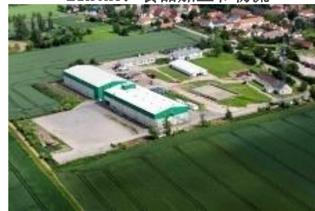
Leipzig: warehouse for grain and farm 莱比锡：粮食仓库和农场
