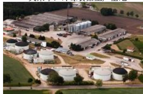
Putlitz: biogas plant and farm 普特利茨：沼气厂和农场
